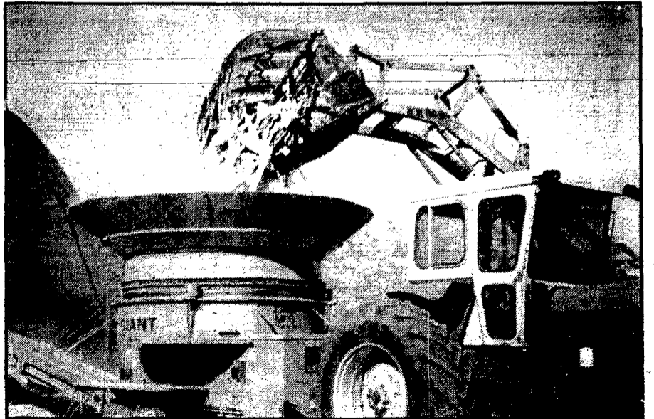
A load of lumber is dumped into the grinder for recycling at Wood Recyclers, located south of Wayne. The Glassmeyers purchased the used grinder from Pennsylvania where recycling has become very popular due to very limited space and state regulations on how and where waste materials can be disposed.
